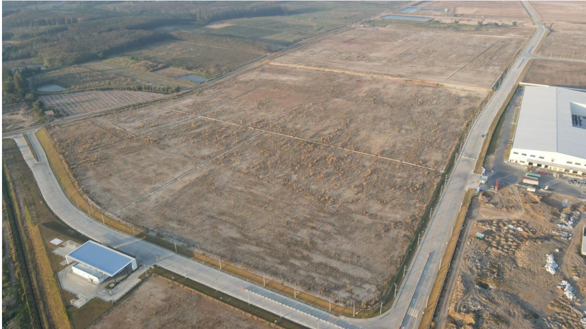
Lotus Bakeries' new production site in the Chonburi Province, Eastern Economic Corridor, Thailand.
